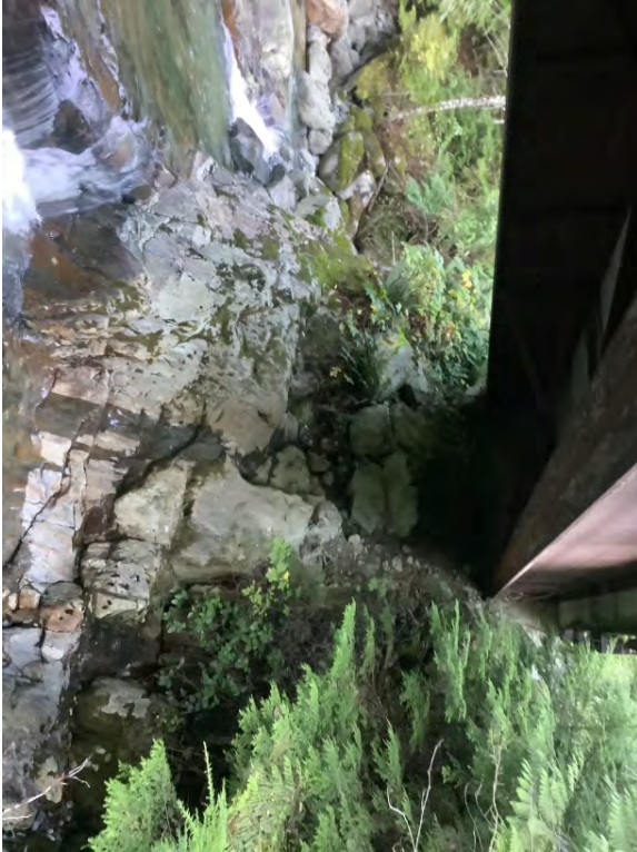
Left Bank Abutment when facing downstream
